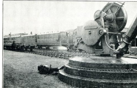
Remove the crane handles before lowering weights by the brake alone.
